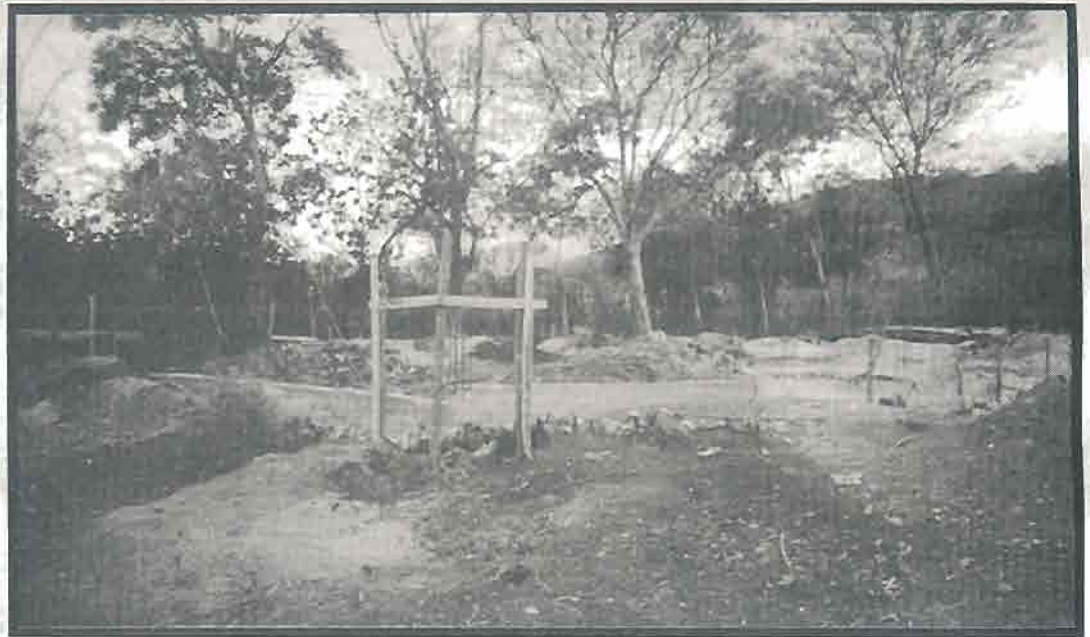
New Church Construction in Pedrenal, Nicaragua
